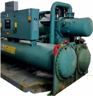
The new central air conditioning unit at Angsana Zhuhai with maglev technology
